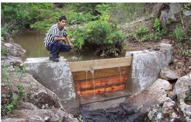
Small dam, Corinto, El Salvador. Photo credit: USAID.
